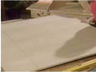
Mark out a 38 inch square
